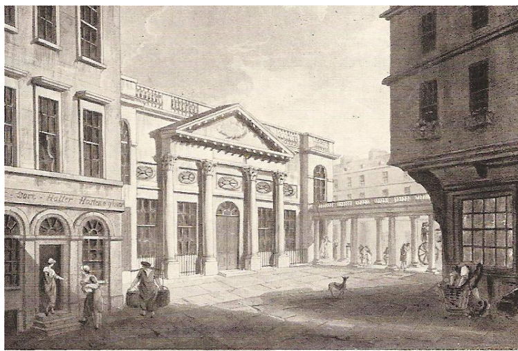
The Portico and Entrance to the Pump Room
